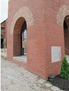
Fig. 1 - Southeast tower, patched and repointed
