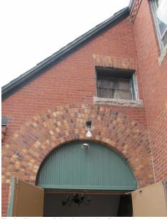
Fig 2 - Entrance following repair of stepped crack
