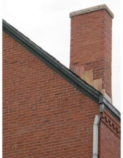
Fig. 3 - Northeast chimney following rebuilding
